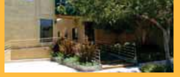
• 136 Main St. - 4757 sq. ft. - Office Building For Sale! 5 Suites, Owner/User Investment, Private underground parking.
